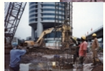
Bored piling works for International Business Park Building 2
