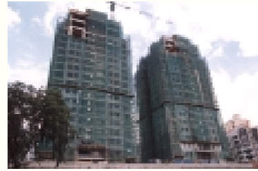
Construction of a commercial and residential complex at Balestier Road
