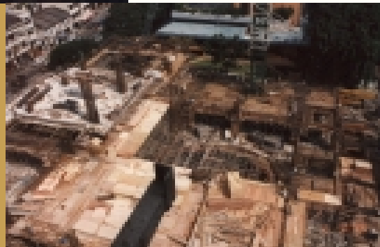
Construction works at Balestier Road
